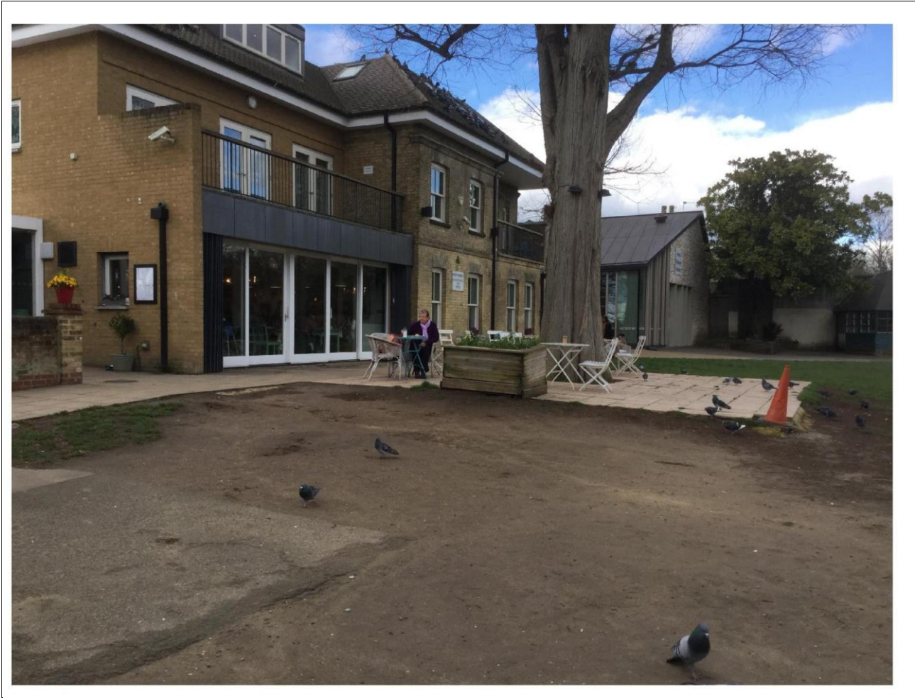
Site photo showing proposed site area
